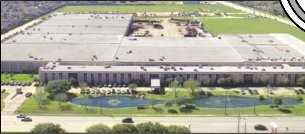
North America Headquarters & Manufacturing Facilities (Houston, TX)
