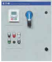
DG1 Enclosed Drive
