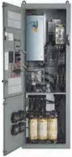
Enclosed 18-Pulse Drive
