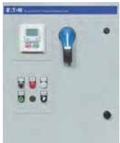
DG1 Enclosed Drive
