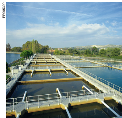
Water treatment application
