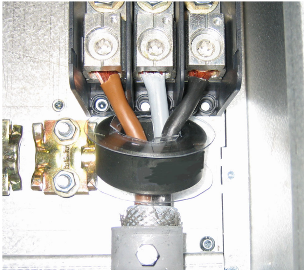
Fig. 55 Ferrite core mounted on the motor cables
