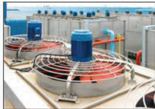
Fans and water pumps
