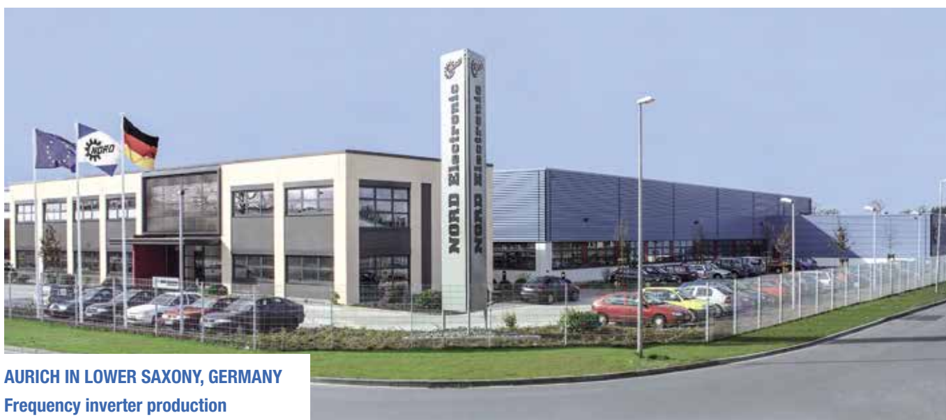
HEADQUARTERS OF GETRIEBEBAU NORD BARGTEHEIDE NEAR HAMBURG, GERMANY Research and development, logistics centre
