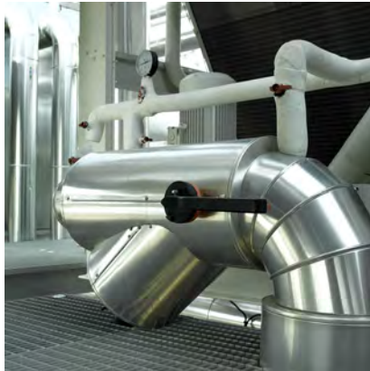
Air conditioning application
